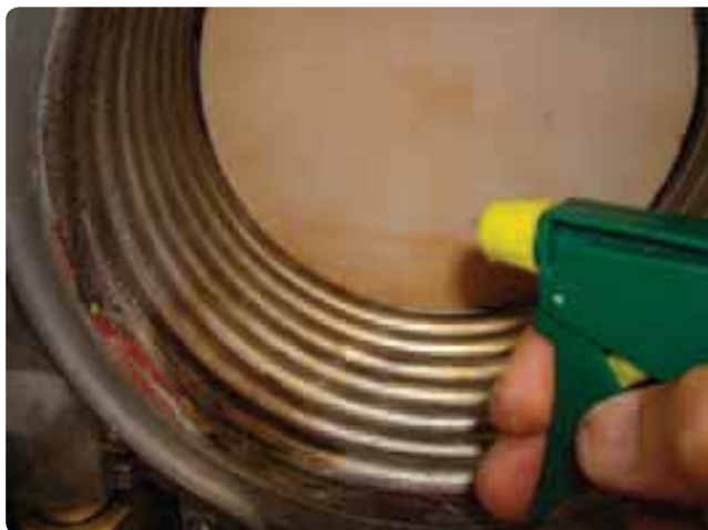
Figure 143 Cleaning the heat exchanger
