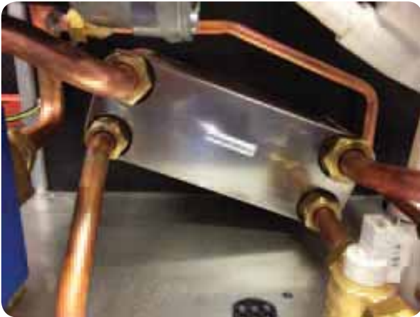
Figure 153 Removal of flat plate heat exchanger by loosening the four fittings. Combi-155
