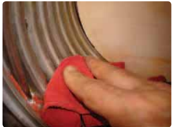
Figure 145 Cleaning the heat exchanger
