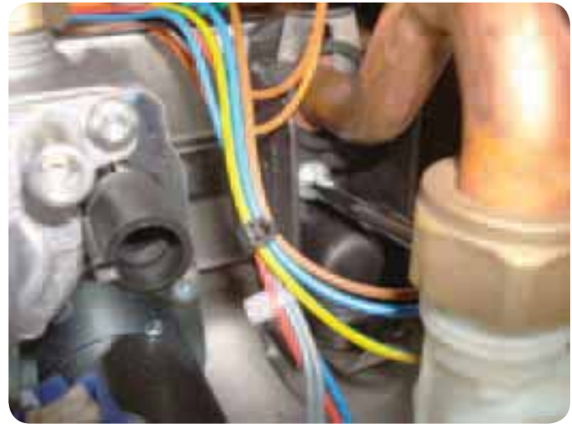
Figure 151 Removal of flat plate heat exchanger (screw on right side) (Combi Only 80/120 shown)
