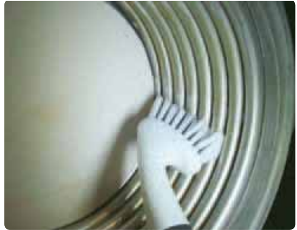
Figure 144 Cleaning the heat exchanger
