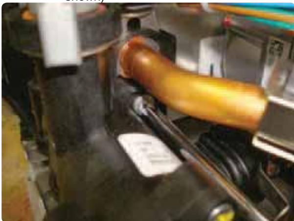
Figure 150 Removal of flat plate heat exchanger (screw on left side) (Combi Only 80/120 shown)
