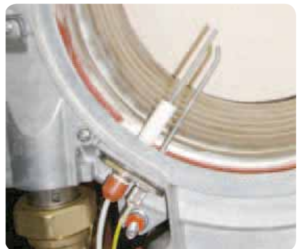
Figure 134 Inspecting ignition electrode
