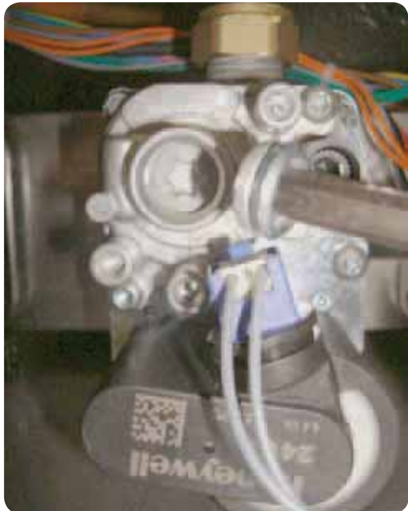
Figure 101 Remove T-40 cover cap with supplied Torx wrench for adjustment
