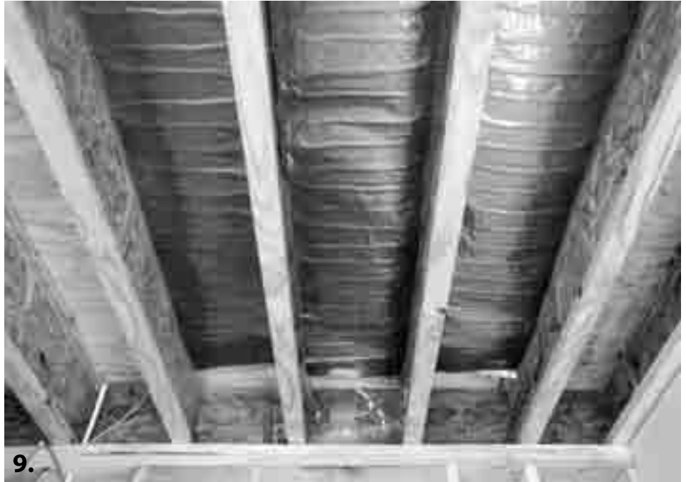
9. Using the same techniques, staple up all other mats.
