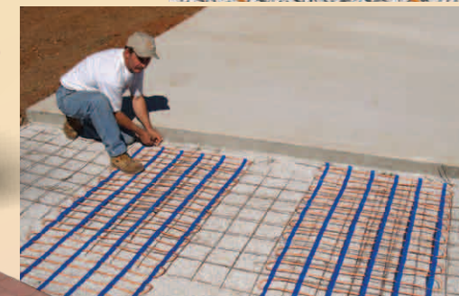
ProMelt Mat in a concrete slab
