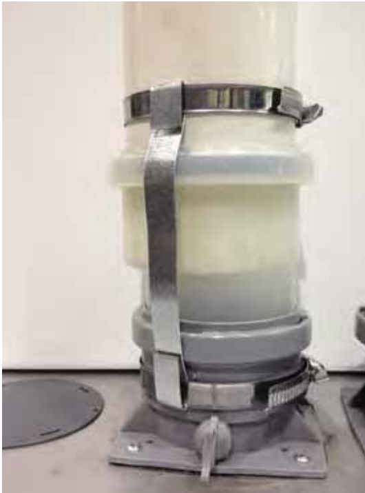
Figure 42 Clamps installed on a PVC pipe going over the PVC adapter
