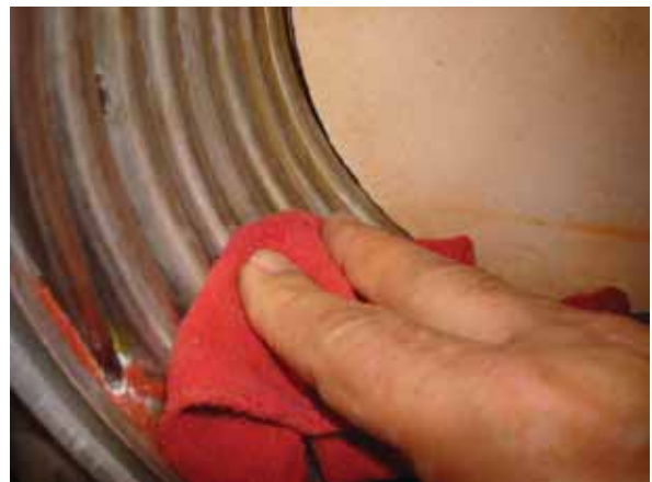
Figure 139 Cleaning the heat exchanger
