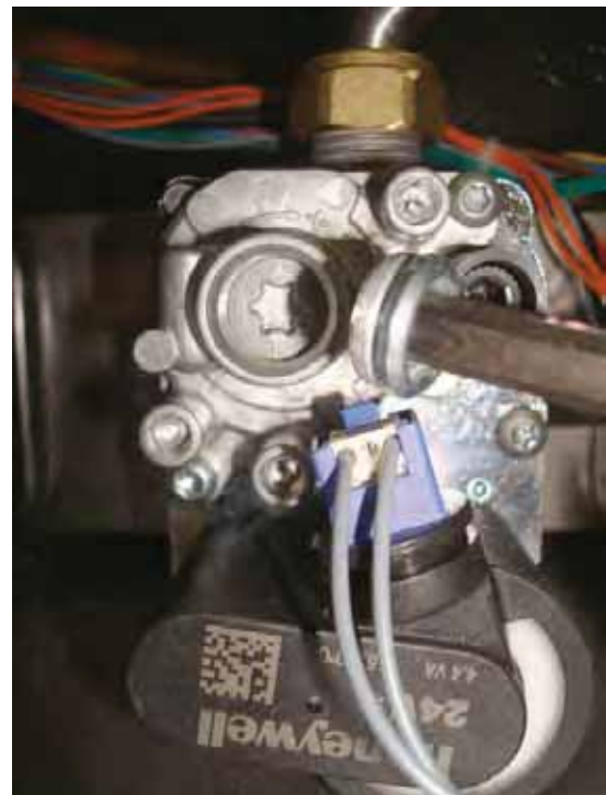
Figure 96 T-40 cap removed for adjustment
