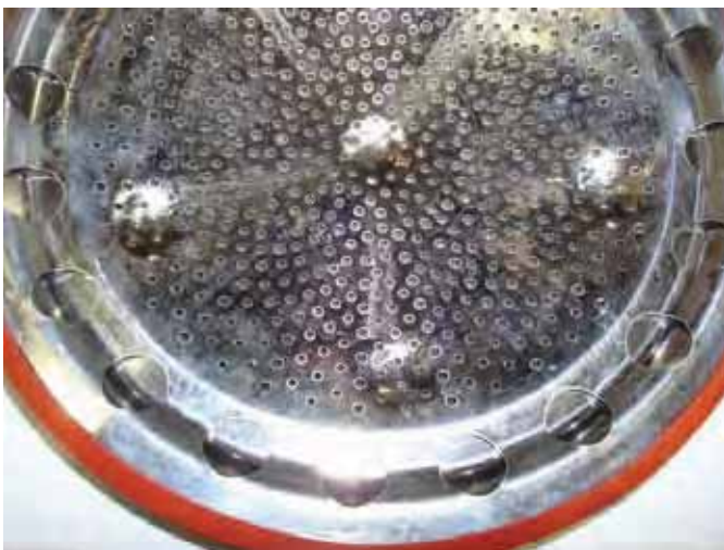
Figure 134 Inspecting interior and cleaning the burner
