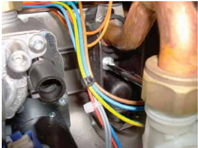
Figure 145 Removal of flat plate heat exchanger (screw on right side)
