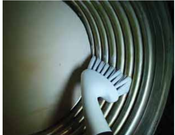
Figure 138 Cleaning the heat exchanger
