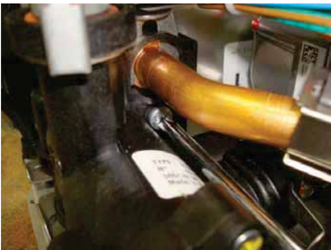
Figure 144 Removal of flat plate heat exchanger (screw on left side)
