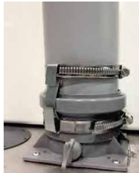
Figure 41 Clamps installed on polypropylene pipe
