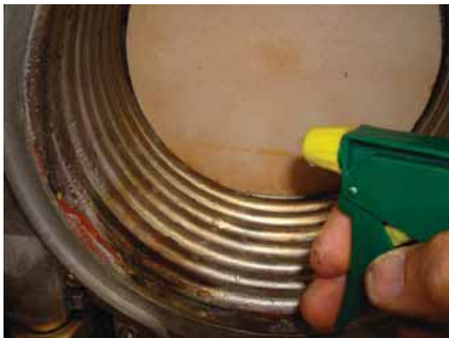
Figure 137 Cleaning the heat exchanger
