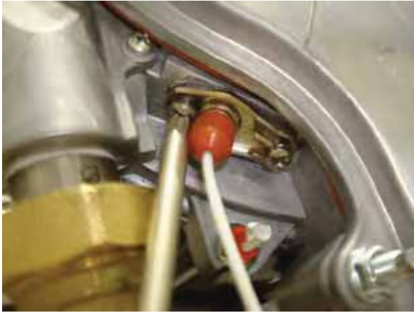
Figure 129 Removal of Ignition electrode
