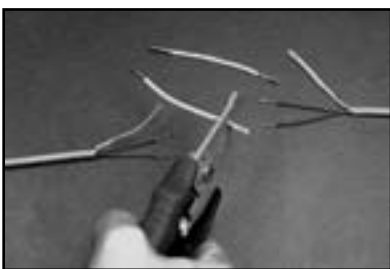
Step 2.10. Remove ½" of the insulation from both ends of the jumper wires.
