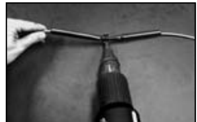
Step 2.18. Slide the outer shrink tube over the entire connection, centering it. Use a heat gun to shrink the tube, beginning near the middle, moving back and forth until it is fully shrunk down. Do not over heat the tube or the heating cable jacket, causing damage. Allow to cool.
