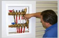
"The Caleffi twist-top actuators save my dealers a lot of time. Individual loops can be purged and filled without taking off all the actuators. Plus the pop-up indicator makes it a cinch to determine if a loop is switched on."
