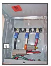
**6.** Lift cover. Remove internal cover plate screw and internal cover. Remove the knock out in the lower right corner of the external connection box. From the rear of the connection box, feed wires, 4-pin and 2-pin plugs into box. Slip the lock nut over wires and plugs and tighten securely onto conduit coupling. Using appropriate fasteners, mount external connection box over pre-drilled hole to fully conceal the hole. Seal around the hole and conduit with silicone caulk from both
