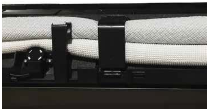
Figure 24: L-bracket Closed (Appearances Will Vary Depending on Indoor Unit Model).
