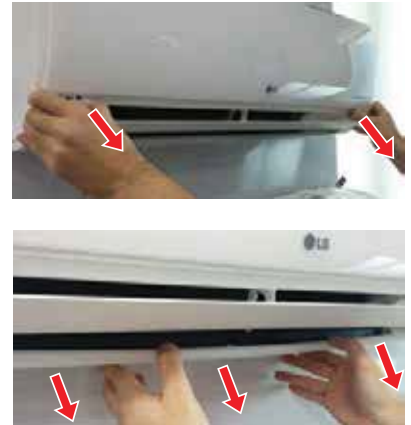
Figure 45: Removing the Bottom Cover, Alternate View.
