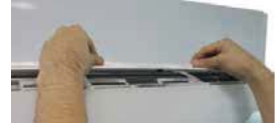
Figure 84: Disassembling the Air Filter (Appearances Will Vary Depending on Indoor Unit Model).
