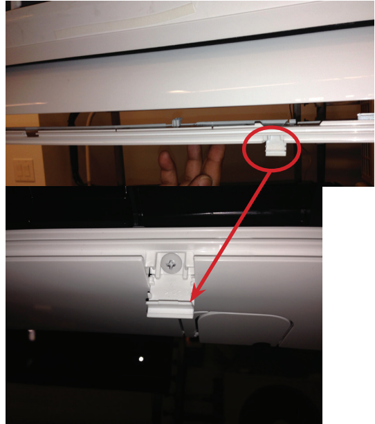
Figure 44: Latch over Screws on Bottom Cover, Indoor Unit.
