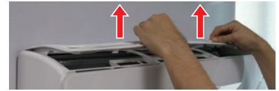
Figure 128: Assembling the Air Filter (Appearances Will Vary Depending on Indoor Unit Model).
