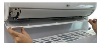
Figure 126: Checking that All Attachment Locations Are Secure (Step 5).
