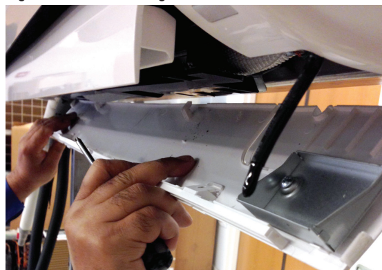
Figure 102: Reattaching the Bottom Cover.
