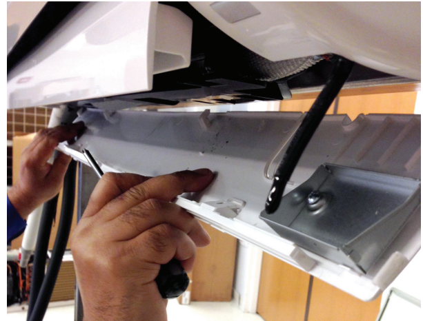
Figure 118: Aligning the Bottom Cover.
