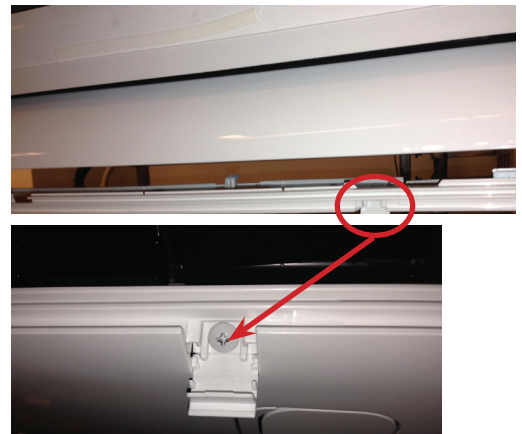
Figure 99: Indoor Unit Knockout (Communication Wires).
