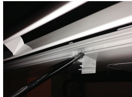
Figure 120: Installing the Screws on the Bottom Panel.
