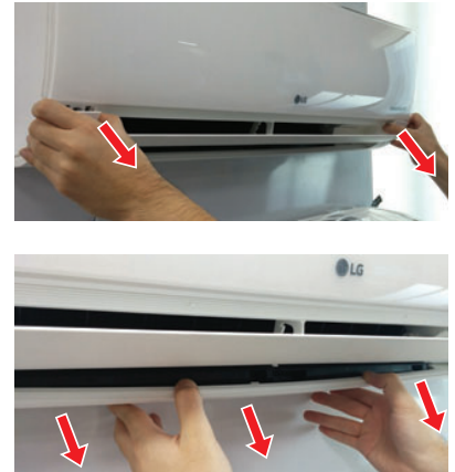
Figure 51: Removing the Bottom Cover, Alternate View.
