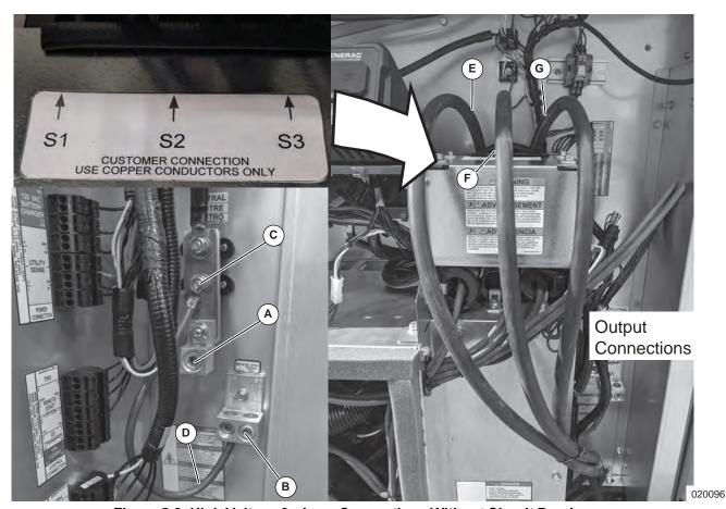
Figure 5-2. High Voltage 3-phase Connections Without Circuit Breaker
