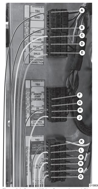
Figure 5-3. Control Wiring Connections - 1-Phase
