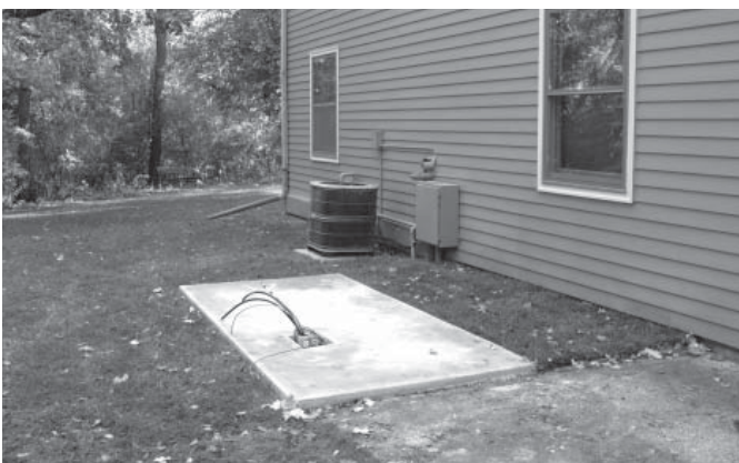
Figure 1.1 — Mounting Pad
