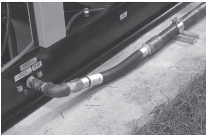
Figure 1.8 — Flexible Fuel Line
