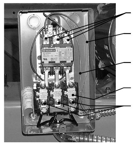
CONNECT INCOMING POWER WIRES TO STARTER TERMINALS L1, L2, L3
