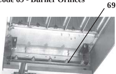
Code 68 - Manifold with Orifices Code 69 - Burner Orifices
