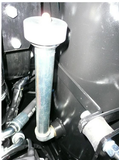
Figure 10.1-1 Checking the oil level in the compressor
