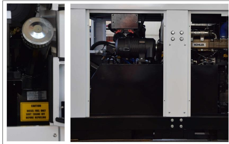
Figure 10.1-2 Fuel tank for Diesel engine
