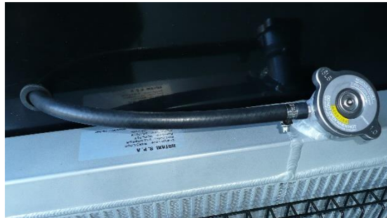
Figure 13.4-3 Checking the coolant radiator
