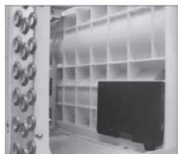
Figure A – Vent (Left side of unit)
