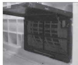
Figure B – Vent Filter Removal
