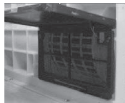
Figure B – Vent Filter Removal
