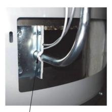
POSITION PILOT TUBING AND IGNITER/SENSOR WIRE
