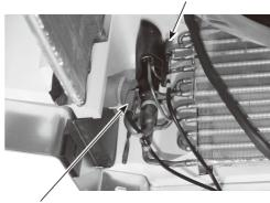
Pipe temperature/liquid thermistor (TH2)
