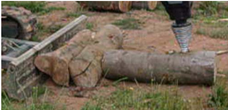
Figure 12: Logs in front of the excavator guard to protect against impact
