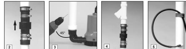
valve. Drill the hole at a 45° angle toward the bottom of the sump to avoid splashing water outside the sump pit. If a 3/16" hole is not drilled in the pipe above the pump, an air lock may prevent the pump from operating.
