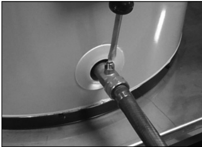
Draining the old water heater.
