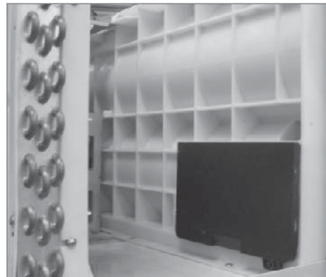
Figure A – Vent (Left side of unit)
