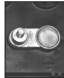
NEGATIVE POST HAS SMALLER DIAMETER
