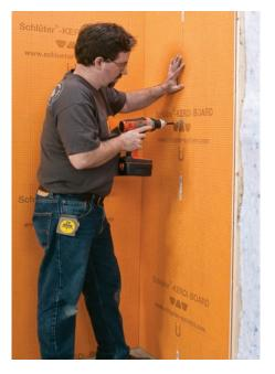
The boards are simply cut to size with a utility knife. The gridlines, which are printed on the surface, are helpful for neat and quick cuts and installation.
