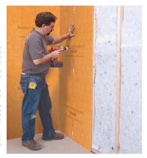
for installation on wall framing with studs spaced at 24" (610 mm) o.c. is 3/4" (19 mm). The maximum recommended on-center fastener spacing is 12" (30.5 cm).
