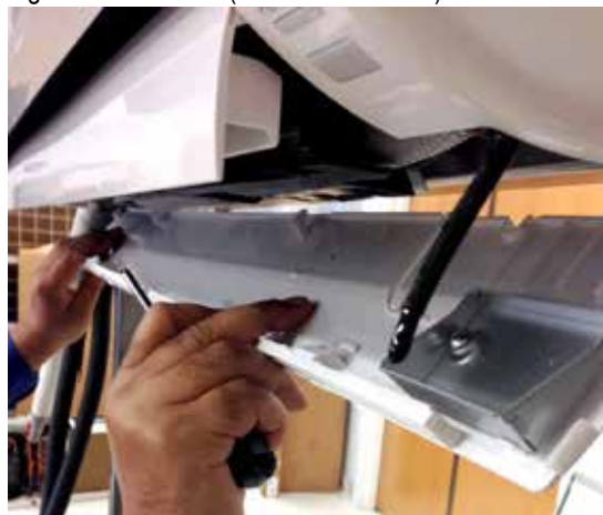
Figure 59: Remove (and Reattachment) Bottom Panel
