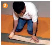
Comb additional unmodified thin-set mortar over the joint using a 1/4" x 3/16" (6 mm x 5 mm) V-notched trowel or the Schluter®-KERDI trowel, which features a 1/8" x 1/8" (3 mm x 3 mm) square-notched design. Using the flat side of the trowel, firmly press the 5" (127 mm)-wide Schluter®-KERDI-BAND into the mortar to ensure 100% coverage and to remove excess mortar and air pockets.
