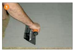
Using a thin-set mortar that is suitable for the substrate, apply the thin-set mortar (mixed to a fairly fluid consistency, but still able to hold a notch) using a 1/4" x 3/16" (6 mm x 5 mm) V-notched trowel, 5/16" x 5/16" (8 mm x 8 mm) V-notched trowel, or the DITRA trowel, which features a 11/64" x 11/64" (4.5 mm x 4.5 mm) square-notched design.
