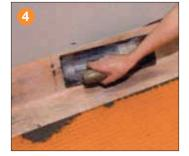
At all wall junctions, apply a 10" (254 mm)-wide strip of KERDI-BAND as described in steps 1-3, centered where the wall and floor meet.
