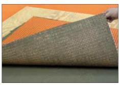
Lift up a corner of the matting to check coverage. Proper installation results in full contact between the fleece webbing and the thin-set mortar. Simply abut end and side sections of adjacent sheets.
