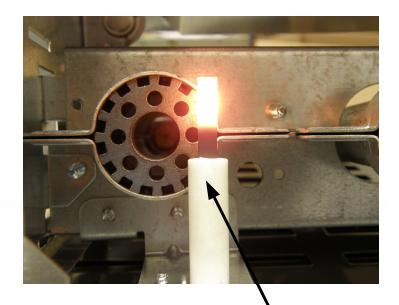
Igniter slightly overlapping OD of burner Correct positioning of ignitor.
