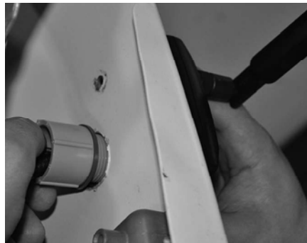
Figure 3.11 - Attaching Mobile Link unit to Fitting
