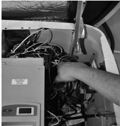
Figure 3.4 - Checking Wire Clearance
