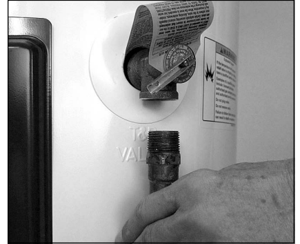
Figure 12 - Removing the T&P Relief Valve discharge pipe.
