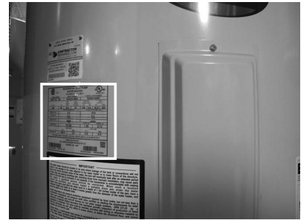
Figure 22 - The water heater’s electrical requirements can be determined from the data plate.
