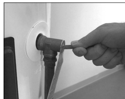
Figure 45 - T&P Relief Valve
