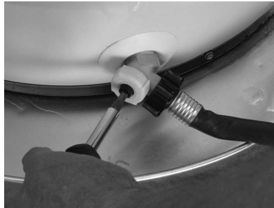
Figure 11 - Draining the old water heater.
