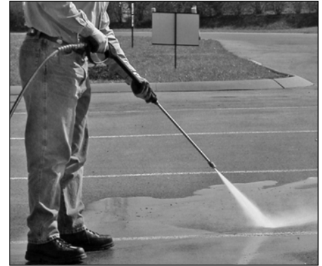
Figure 14 - Optimum angle to cleaning surface
